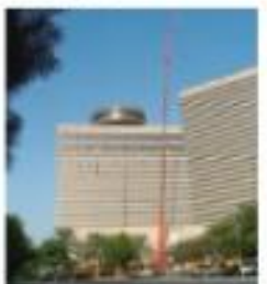
2010 Chiller lift Dubai Hayat Regency
