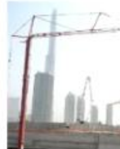
2008 Downtown Construction Dubai
