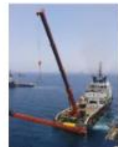
2011 Flare Boom Installation Dubai
